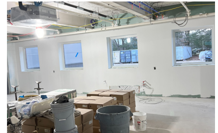
Above: Painted 1st floor classroom stocked with floor tile
